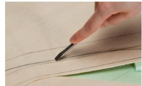
**Installing contact wire:** Press the contact wire into the groove with a flat head screwdriver or joiner, ensuring it is correctly seated in the groove.
